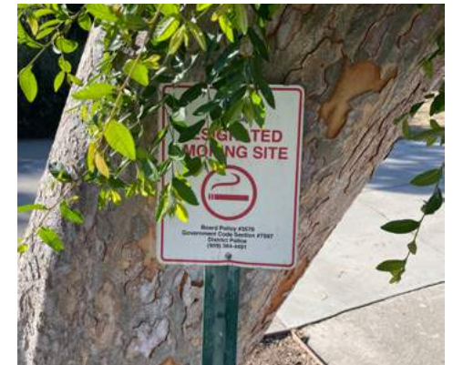
OBSTRUCTED SAFETY SIGNAGE
