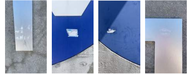
SOME SMALL-SCALE DAMAGE TO SIGNAGE
