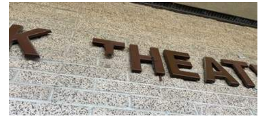
SIGNIFICANT DAMAGE AND MISSING LETTERS ON SOME SIGNS
