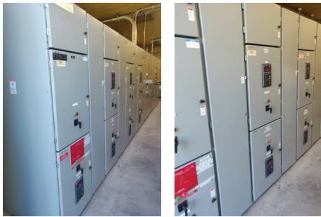
Main Switchgear
