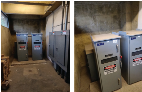
Crafter Center Load Interrupter Switch
