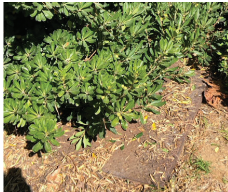
Gas vault on the south side of the gym building
