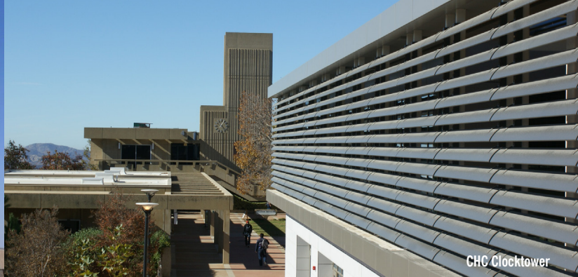
Valley College central plant is equipped with thermal energy storage
