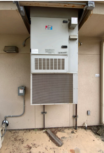
TYPICAL WALL-MOUNTED HEAT PUMP
