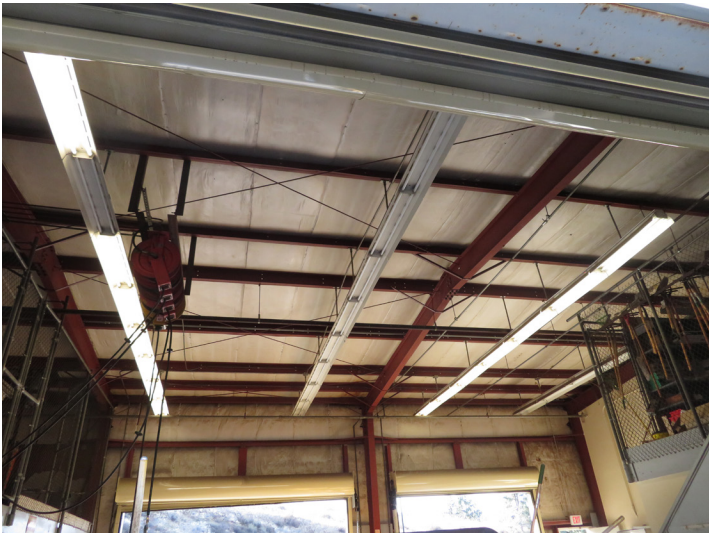
LOW BAY LINEAR FLUORESCENT LIGHT FIXTURES
