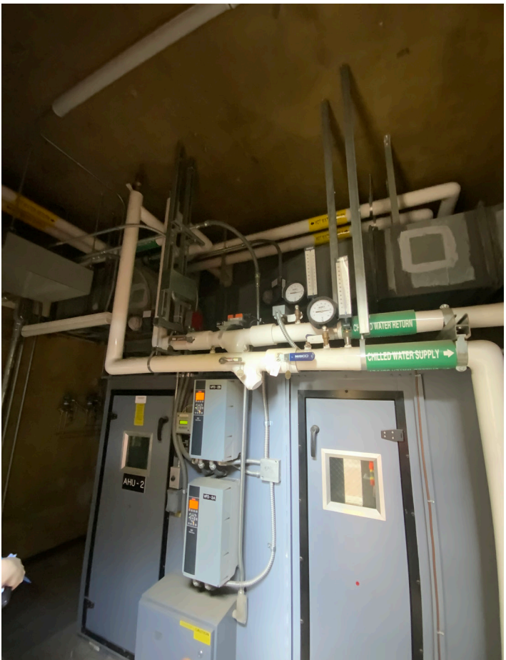
TYPICAL AIR HANDLER UNIT WITH CHILLED WATER CONNECTION
