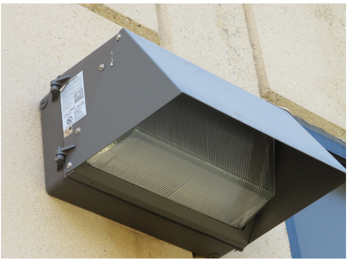
TYPICAL WALL MOUNTED EXTERIOR LIGHTING FIXTURE
