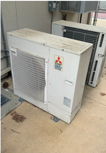
TYPICAL SPLIT SYSTEM CONDENSING UNIT
