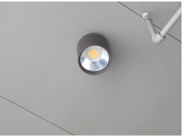
TYPICAL CYLINDRICAL LED LIGHT FIXTURE
