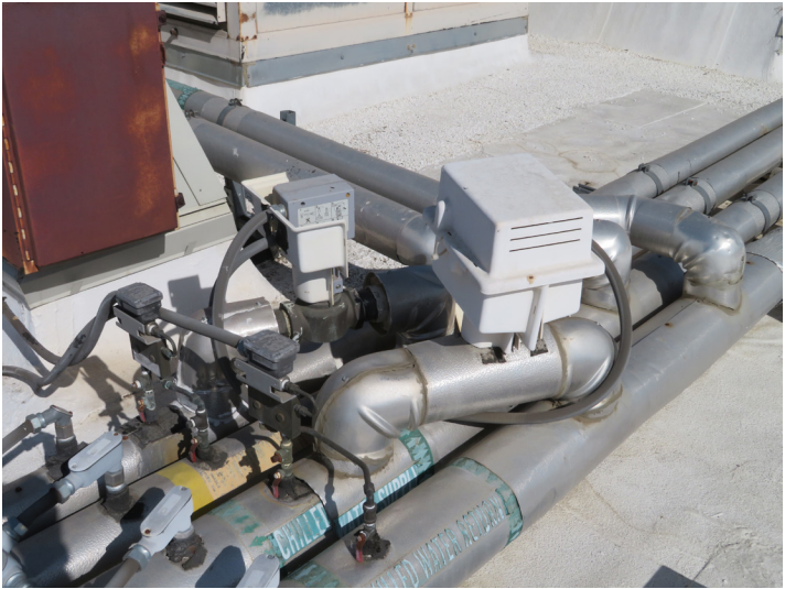
CHILLED WATER CONNECTIONS TO AIR HANDLING UNITS
