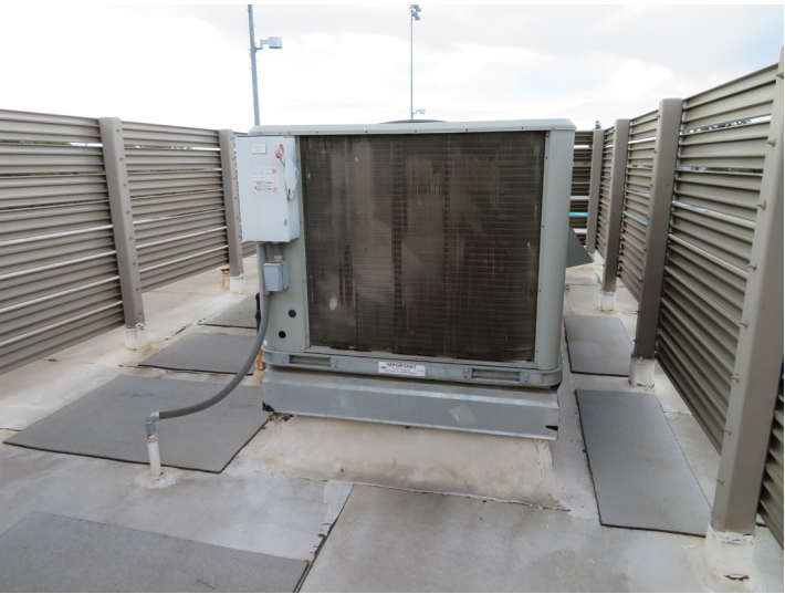
TYPICAL PACKAGED ROOFTOP UNIT
