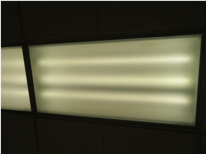
TYPICAL 2'X4' RECESSED TROFFER FIXTURE
