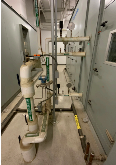
AIR HANDLER UNITS WITH CHILLED WATER CONNECTIONS
