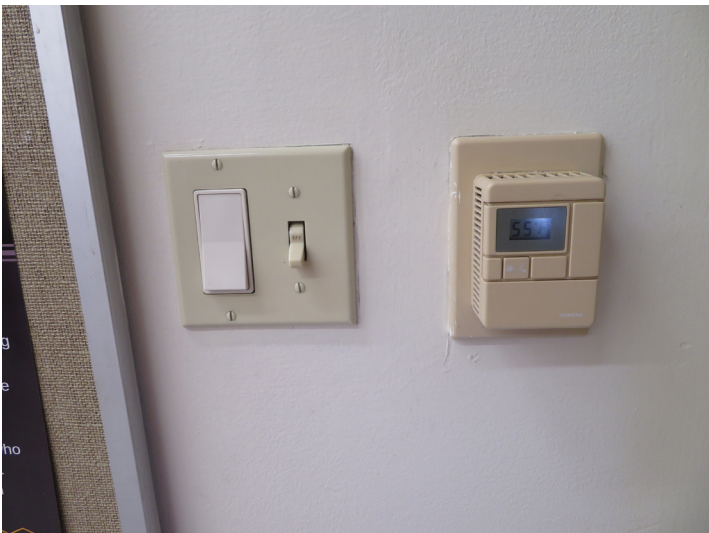
TYPICAL LIGHTING SWITCH AND TEMPERATURE SENSOR
