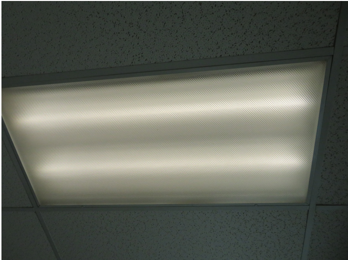
TYPICAL LIGHTING FIXTURE WITH F32T8 LAMPS
