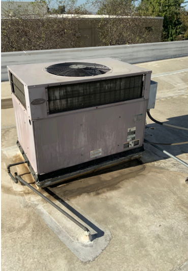
TYPICAL PACKAGED ROOFTOP HEAT PUMP
