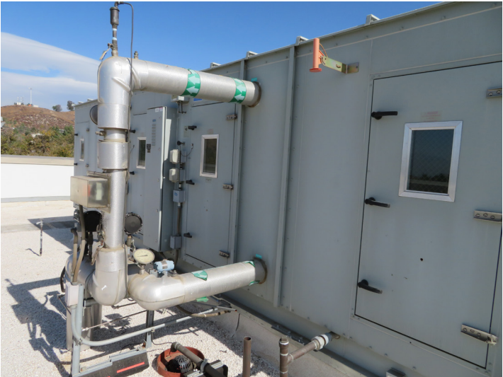
TYPICAL AIR HANDLER UNIT WITH CHILLED WATER CONNECTION
