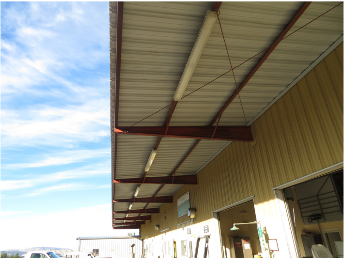
LOW BAY LINEAR FLUORESCENT LIGHT FIXTURES
