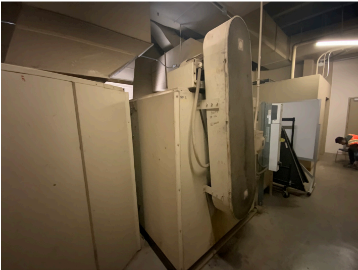
MULTI-ZONE AIR HANDLING UNIT
