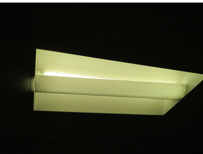
TYPICAL LIGHTING FIXTURE WITH F32T8 LAMP
