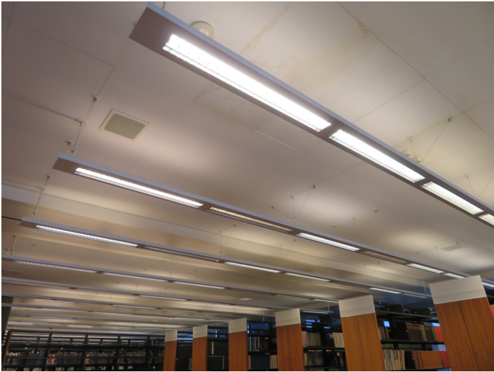
TYPICAL BOOKSTACK 4’ SUSPENDED LIGHTING LAYOUT
