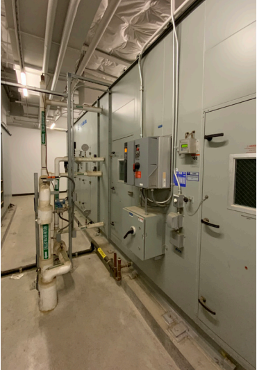
AIR HANDLER UNITS WITH CHILLED WATER CONNECTIONS
