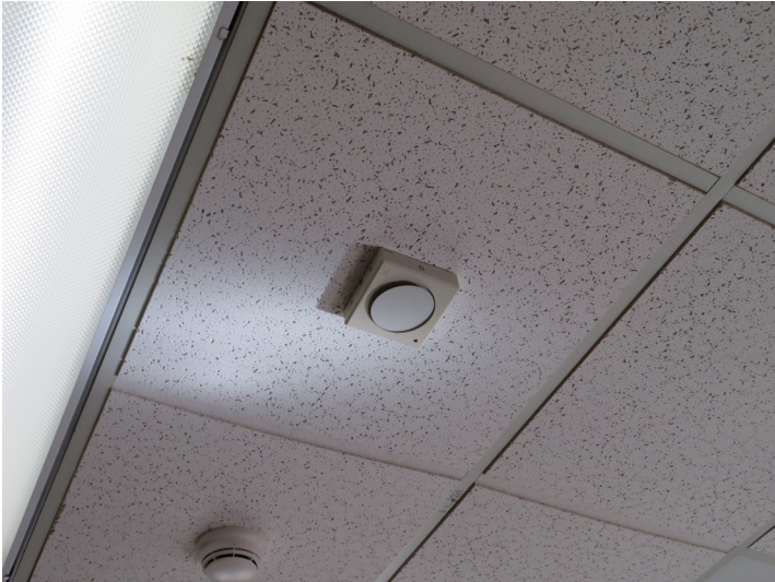
TYPICAL CEILING MOUNTED OCCUPANCY SENSOR
