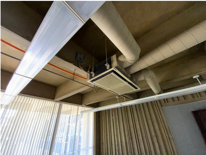
INTERIOR LIGHTING FIXTURE AND OFFICE FAN COIL UNIT
