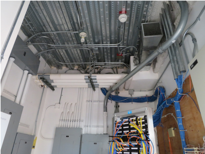
FAN COIL UNIT WITHIN ELECTRICAL ROOM
