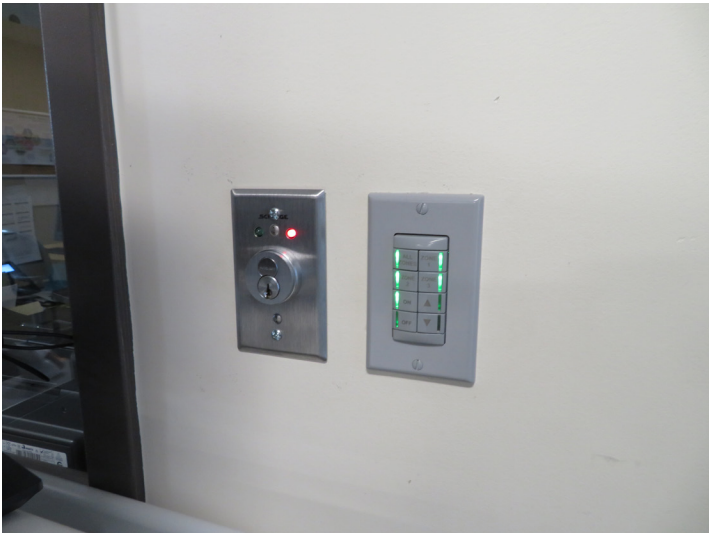
TYPICAL LIGHTING DIMMING CONTROLS FOR CLASSROOM
