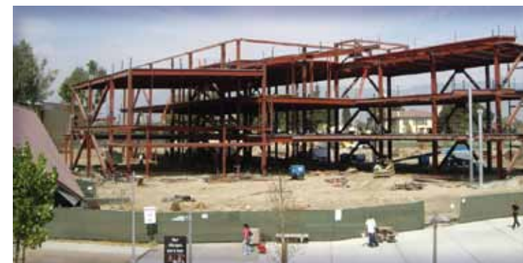
North Hall Steel Framing in Progress
