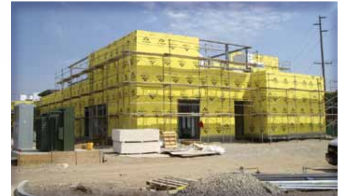
Media/Communications Exterior Wall Sheathing
