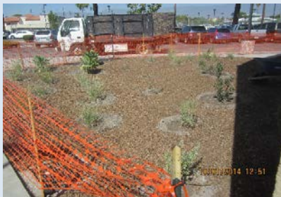
Planting and Mulch Install at North Side of ADSS Building
