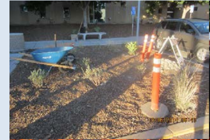
Final work for Landscape around Admin. Bldg.
