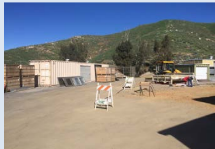
Marking out excavation for footings
