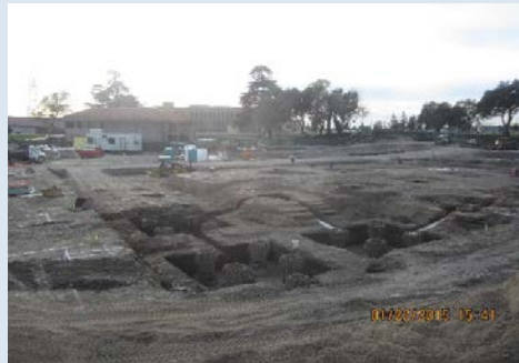
North East Side - Digging Foundations
