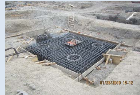
Pile Cap Foundation - Rebar Installation
