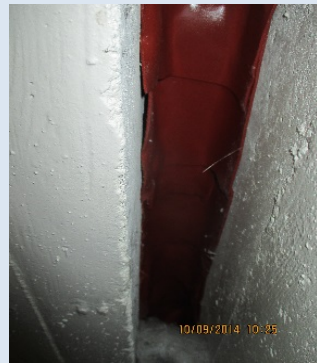
Fire Caulking at Seismic Joint
