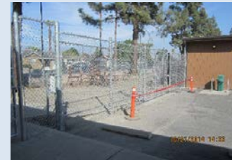
Fencing around Welding Yard
