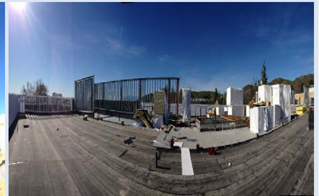
Work Progress at Lab Wing Building
