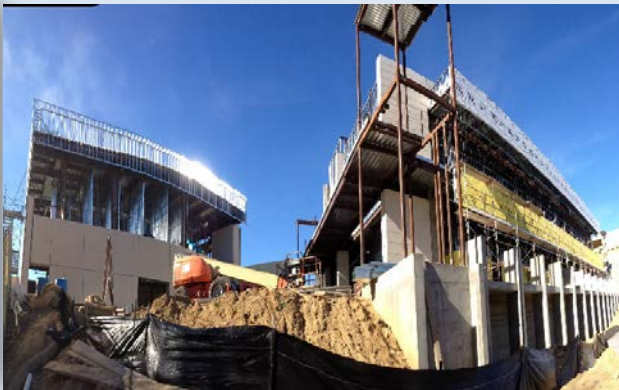
Work Progress at Lab & Lecture Wing Building
