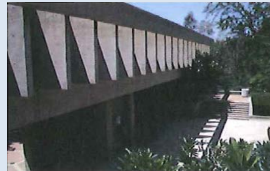
Exterior Photo of 3rd floor offices
