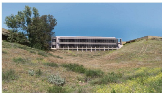
South Elevation - Lab Wing NEW SCIENCE BUILDING | DESIGN DEVELOPMENT - USER MEETING OCTOBER 17, 2012 NTD ARCHITECTURAL Crafton Hills
