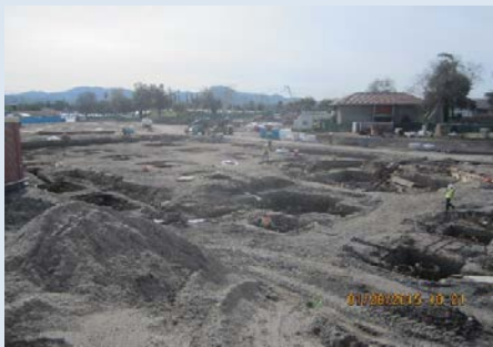
East Side - Digging Foundations
