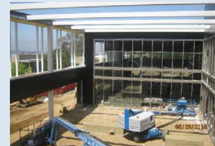
Curtainwalls at Interior Courtyard
