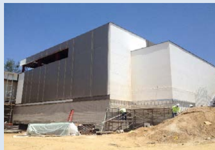
South Elevation With Metal Panels
