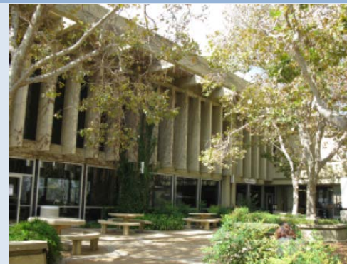
Exterior Building Photo of East elevation
