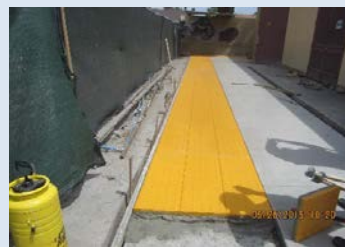
Truncated Dome Installation
