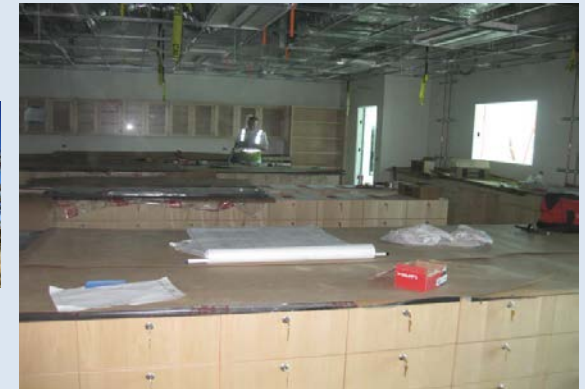
Work Progress at Lab Wing Building
