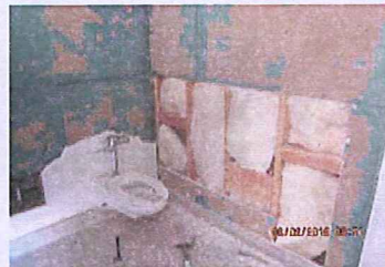
Modular Restroom Upgrades
