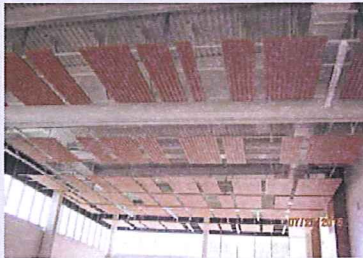
Ceiling at Multi-Purpose Room
