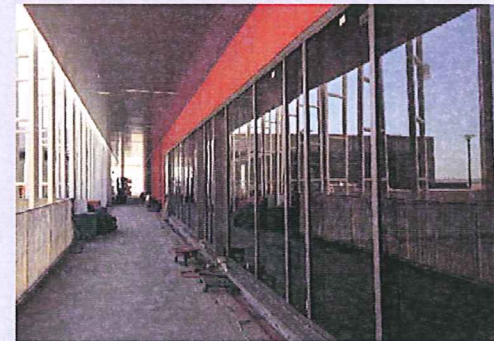
Curtain Wall Installation at 2nd Floor
