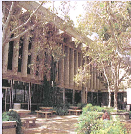
Exterior Building Photo of East elevation
