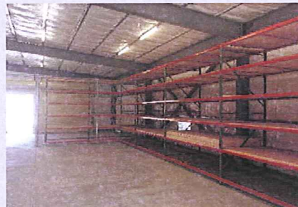
New Racks at New Warehouse
