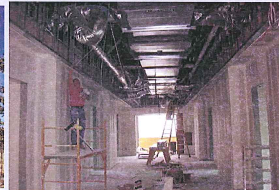
Work Progress at Lab Wing Building
