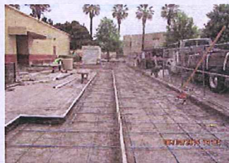
West Side Sidewalk work
