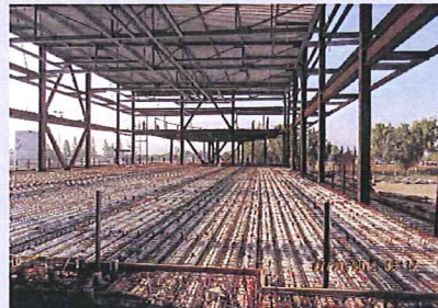
Segment C- Installation of roof decking
