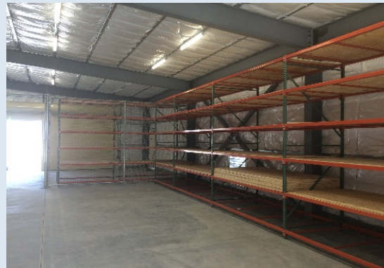
New Racks at New Warehouse
