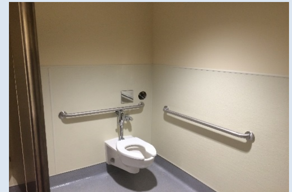
Finishes at New Restroom
