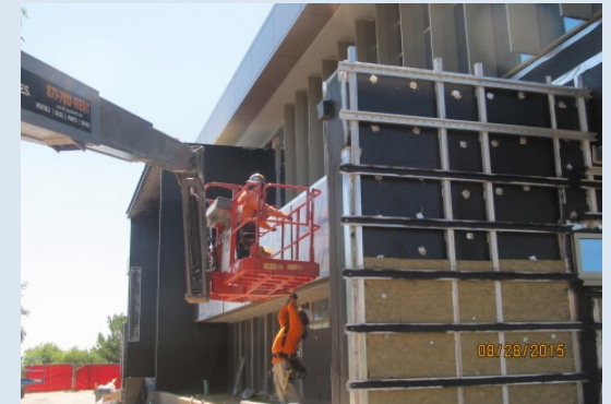
Metal and Fiber Cement Panels at East Elevation
