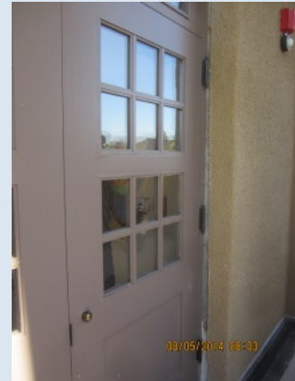
North Exterior Door
