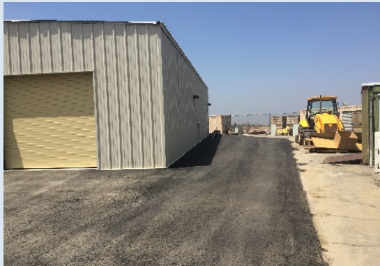
Exterior of New Warehouse
