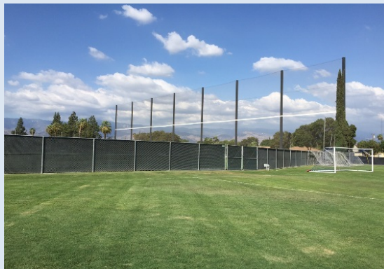
Future location for the netting fence
