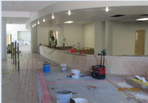
Tile and Casework at Concourse
