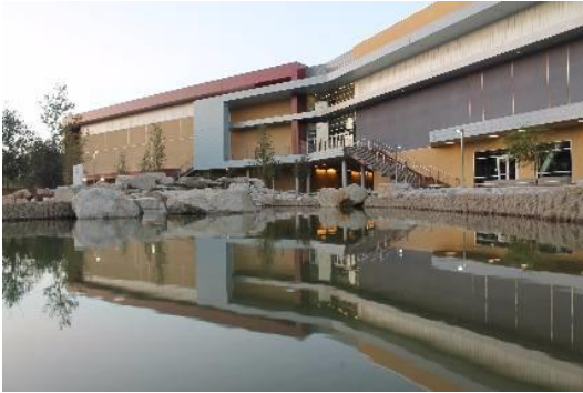
Building Name: Kinesiology & Athletics Complex Campus: San Bernardino Valley College Sustainability: Info pending
