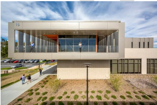
Building name: Public Safety & Allied Health Campus: Crafton Hills College Sustainability: Info pending
