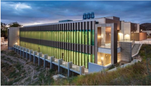
Building name: Canyon Hall Campus: Crafton Hills College Sustainability: LEED Gold Certified
