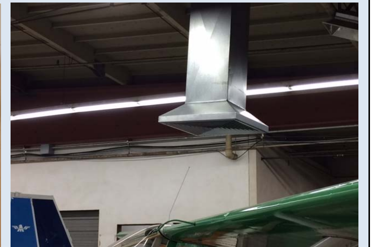
Typical Transition and Diffuser (Aero Lab)
