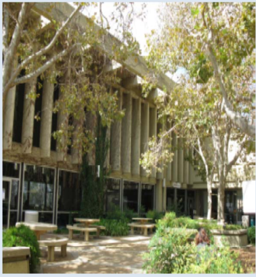
Exterior Building Photo of East Elevation
