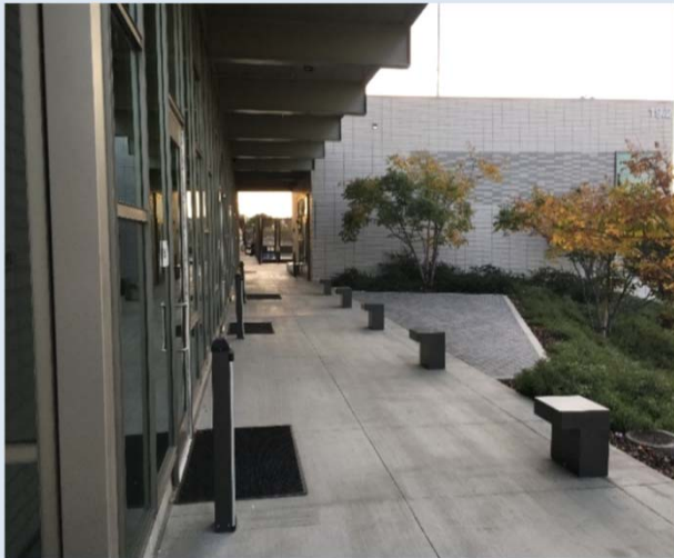
Front of Building
