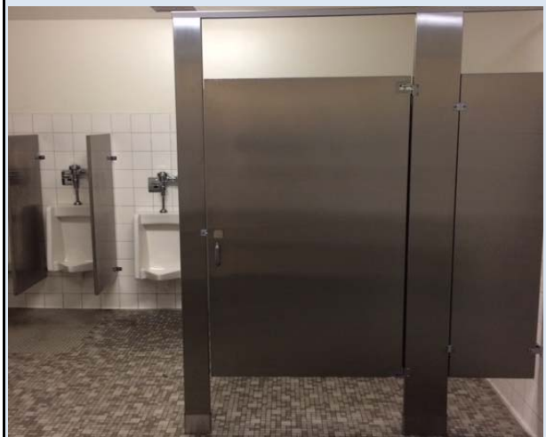
Completed Men's Partition
