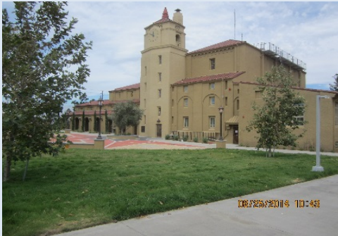
Auditorium South Entrance
