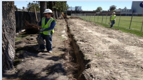
Conduit Trench at Soccer Field
