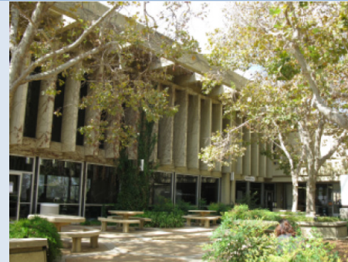
Exterior Building Photo of East elevation
