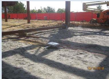
Preparation for Foundations
