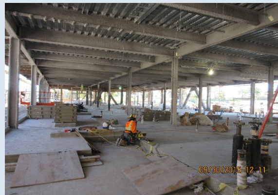
Seg C - Fire Proofing Beams and Columns
