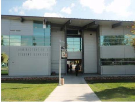
Administration and Student Services Building is a two story building and is used for student services and administration. AD/SS has 26,016 ft<sup>2</sup> of conditioned floor area. The building has insulated corrugated sheet metal envelope with standing seam sheet metal sloped roof. Most of the occupancies are used for office activities. Building is seven years old.
