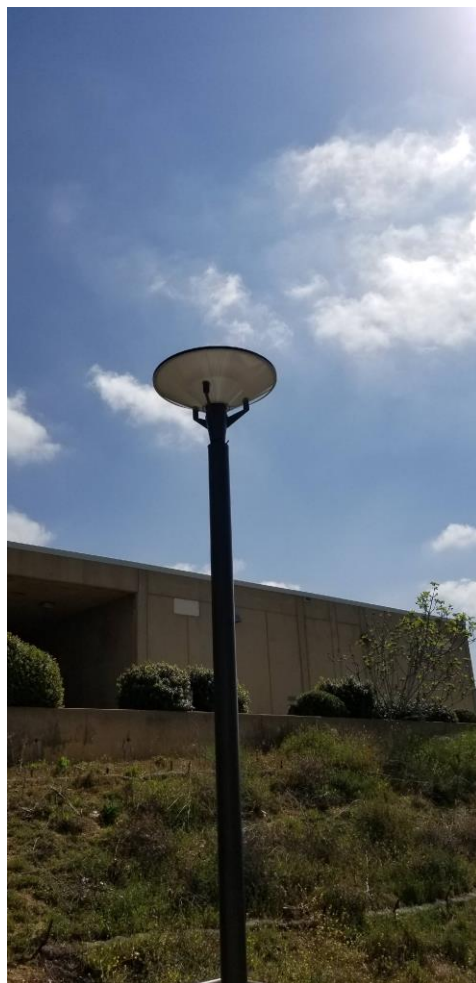
Existing Walkway Post Top – B1
