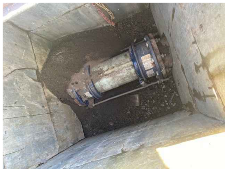
Existing Vault for new PRV
